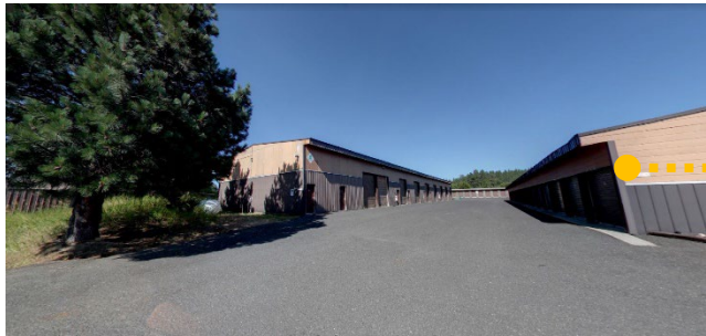
EXISTING STORAGE FACILITY
