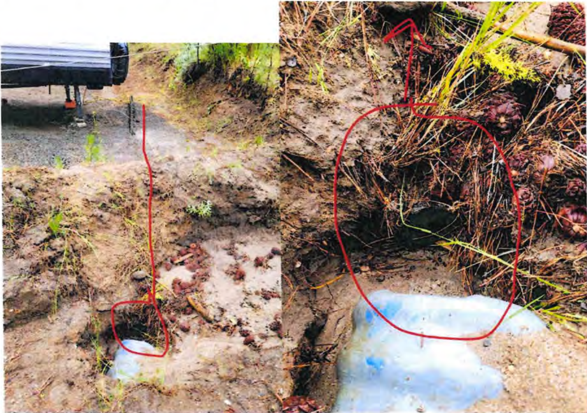
Picture 5 a & b: shows a pipe from an RV pad run to the ditch
