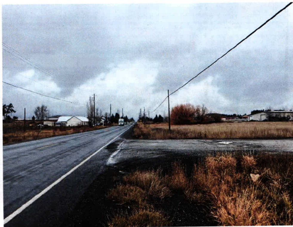
Photo 2 - South of approach looking north (11/20/25)
