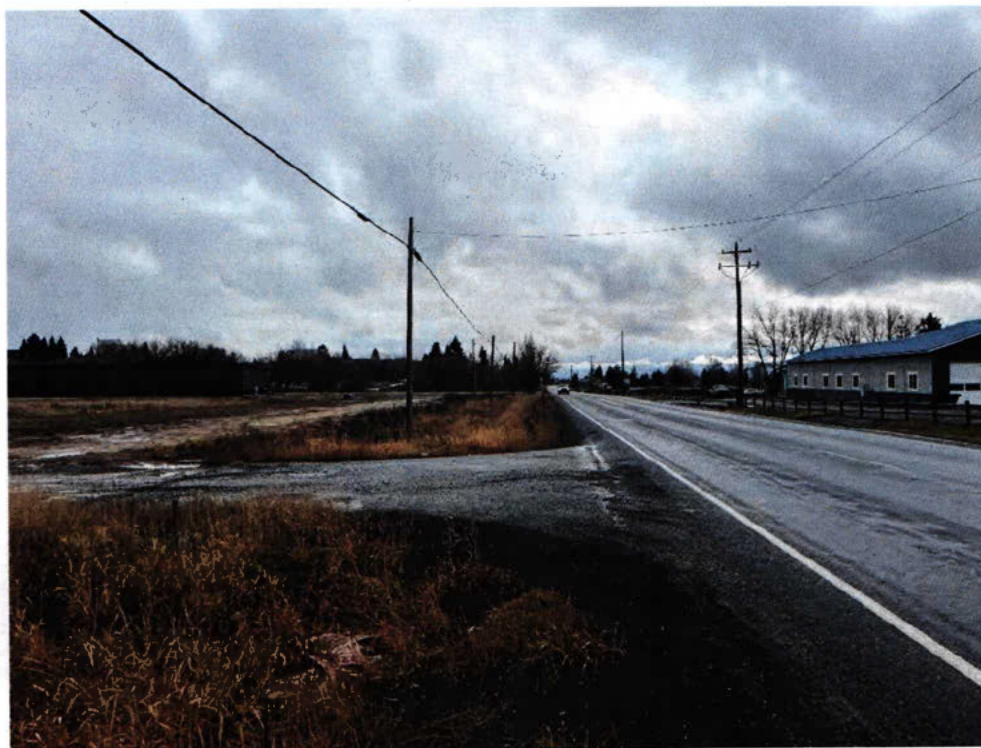
Photo 1 – North of approach looking south (11/20/25)
