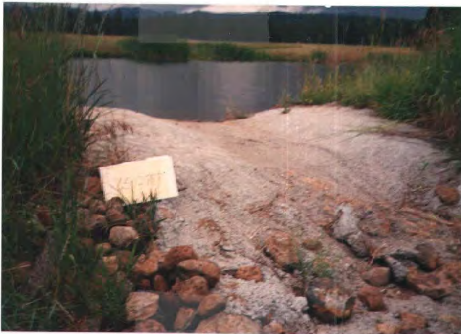
Picture #1 Spillway for dam
