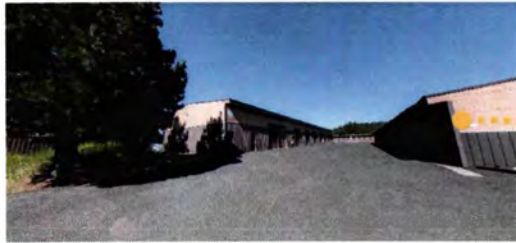
EXISTING STORAGE FACILITY
