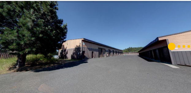
EXISTING STORAGE FACILITY
